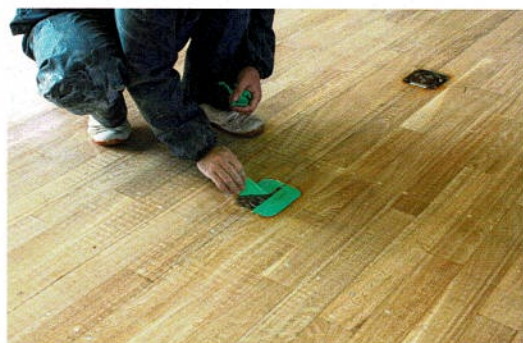
床金具の養生撤去
