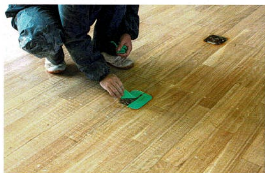
床金具の養生撤去
